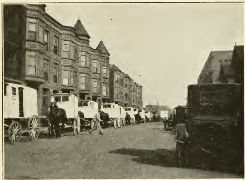
FIGURE 8.—A line of wagons waiting to be checked in at the plant shown in Figure 7
